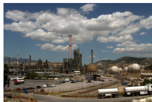
refinery facilities fosR1700006
