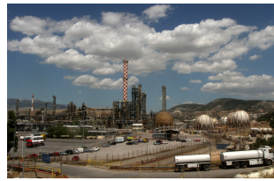
refinery facilities fosR1700006
